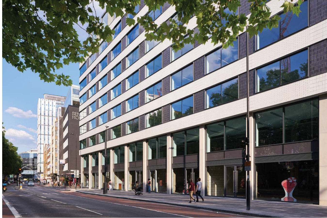
Looking east towards Old Street roundabout with Unit 1 in the foreground.
